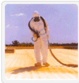
Spray heat insulation
